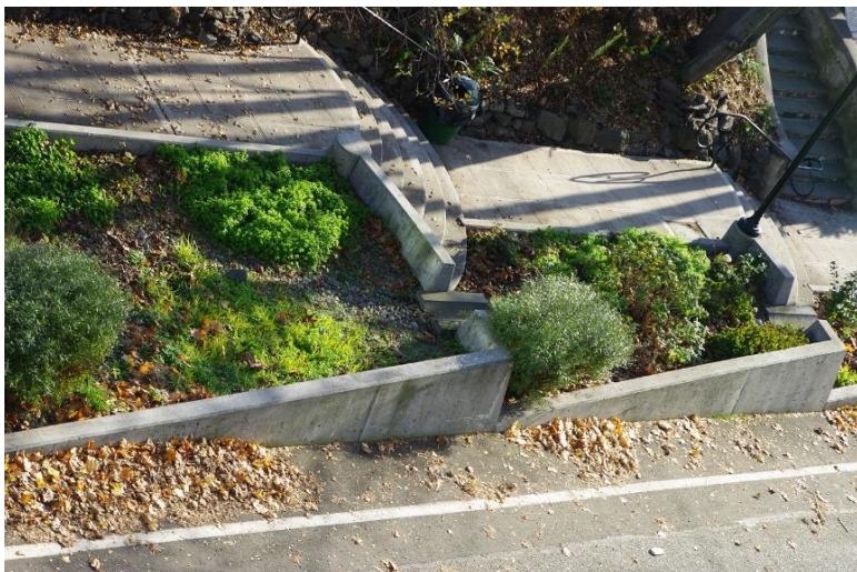
Figur 5. Trappformad sammankoppling av regnbäddar längs Growing Vine Street i Seattle, USA. (The Pennsylvania State University, 2018)
